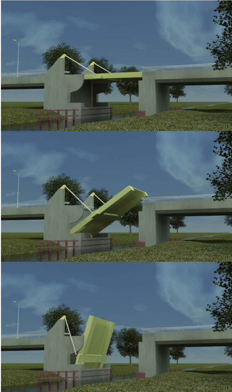
Fig. 7.12 Conceptual design of the Wing-type bascule bridge (Conceptual design together with Gerard Bouwman & Martijn van Dijk, Hollandia, 2012)
